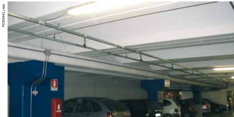
Canalis KBA supplying luminaires nearby sprinklers.
