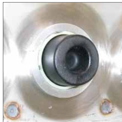
J Insulated blanking plugs are compulsary for sealing off bushings on an energized switchboard.
