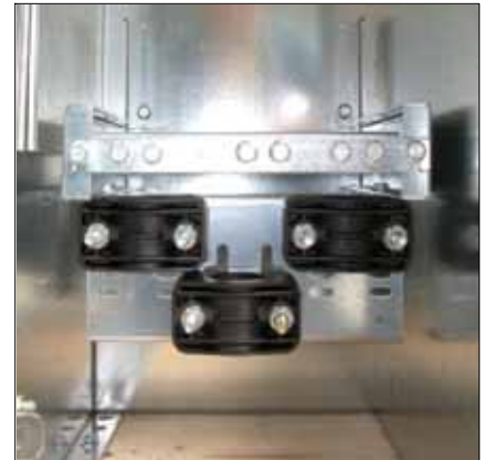
▮ Cable clamp for C function.
