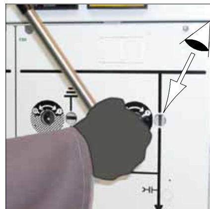
J Lift the lever: The switch is now closed. J Remove the lever.
