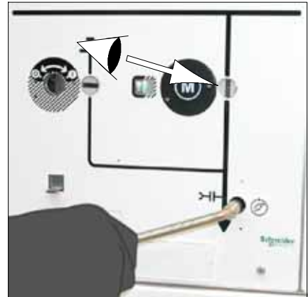
J Continue until the operation is completed (mimic diagram changes). J Remove the crank handle.
