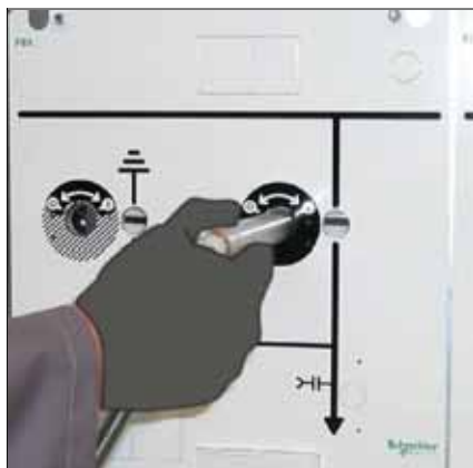
J Insert the appropriate lever (black end) into the load-break switch socket.
