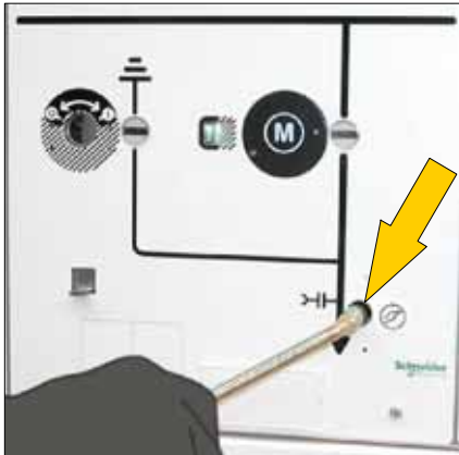
J Insert the backup handle for the switch into its hole.
