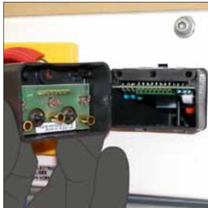
J Extract the voltage indicator unit.
