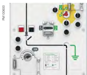
OCO mechanism in D06H unit
